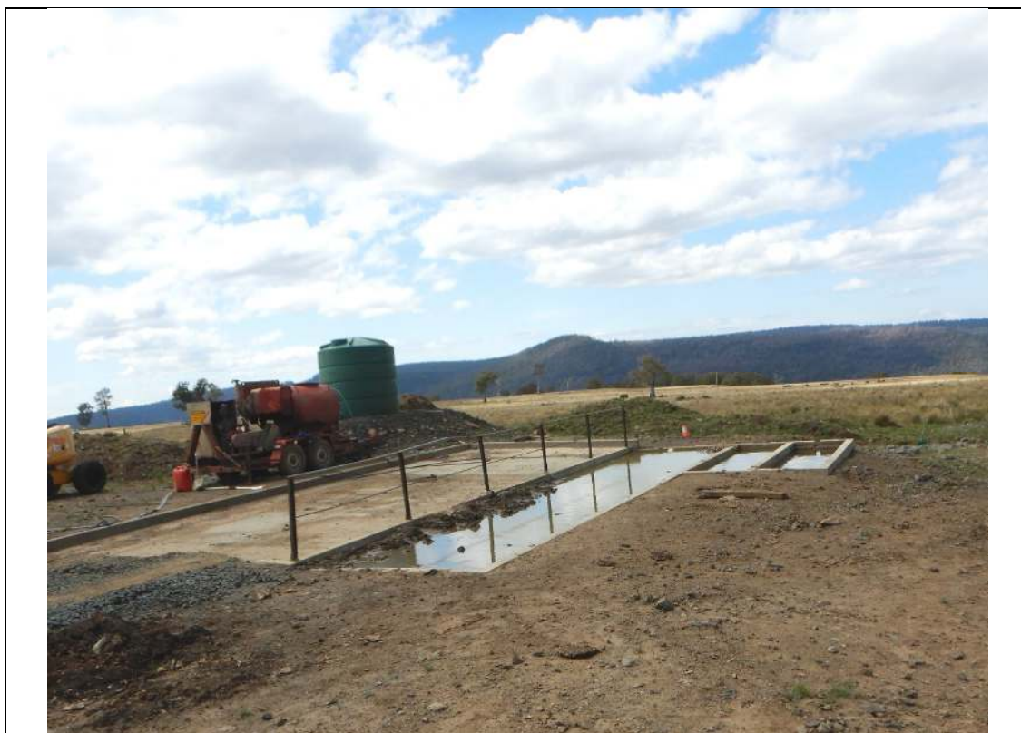
Plate 4.5 – Wash Down Bay at Construction Compound maintained during construction works
