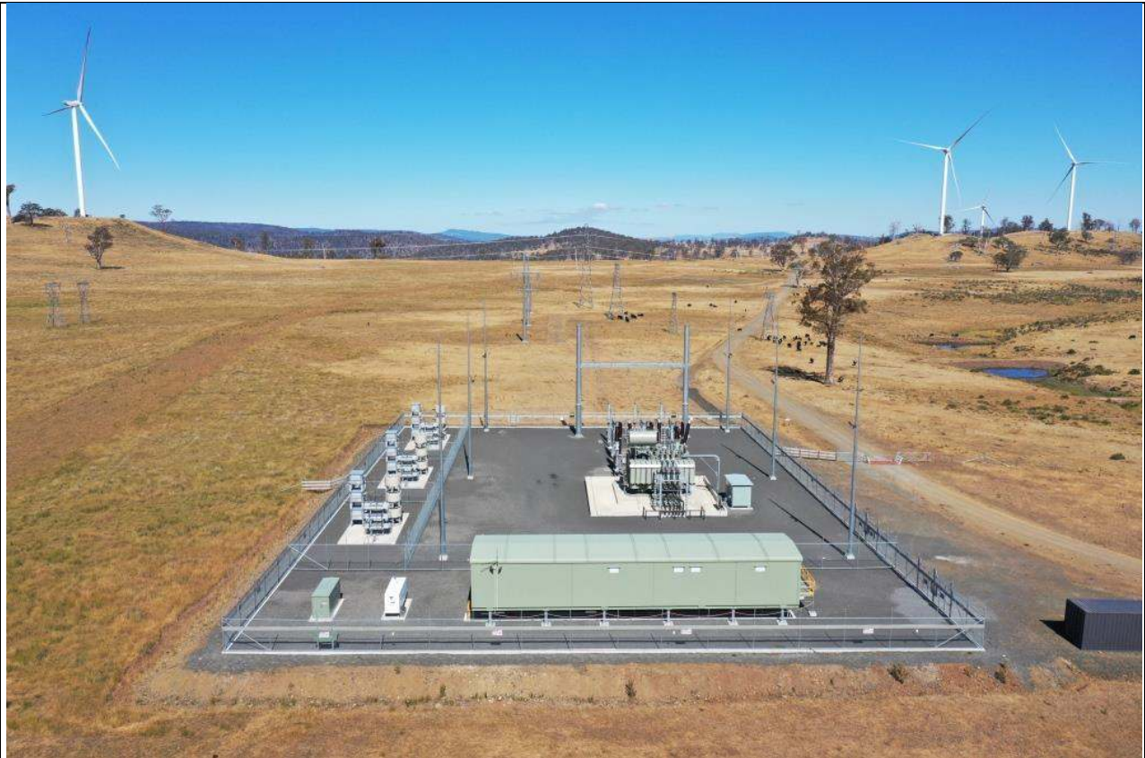
Plate 3.3 – View of installed CHWF 33kV/220kV substation
