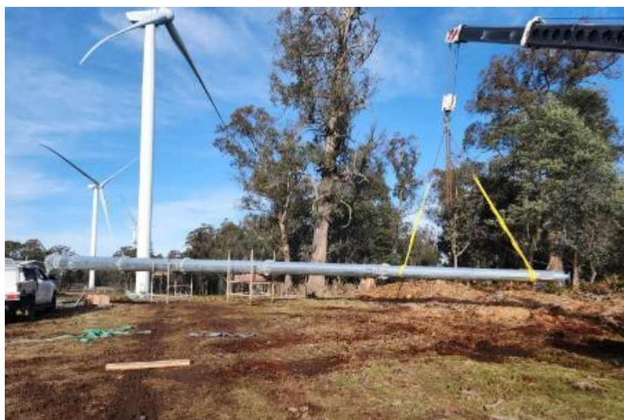
Photograph B4: Lifting the tower
