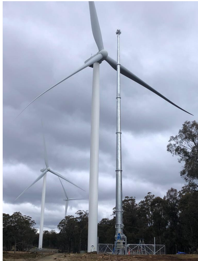
Figure 4.1: New 30m IDF tower installed as mitigation for mortalities at Turbine 46.
