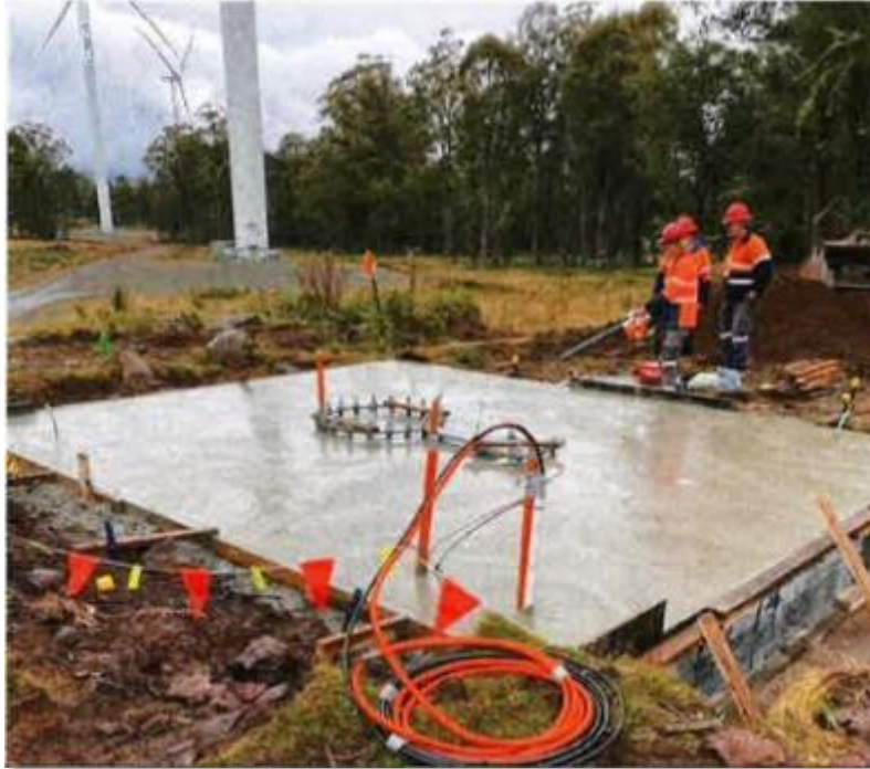
Photograph B1: Foundation for taller tower
