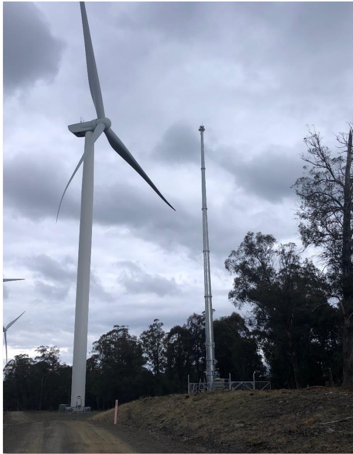
Photograph B5: Installed 30m IDF Tower (IDF 17-45)
