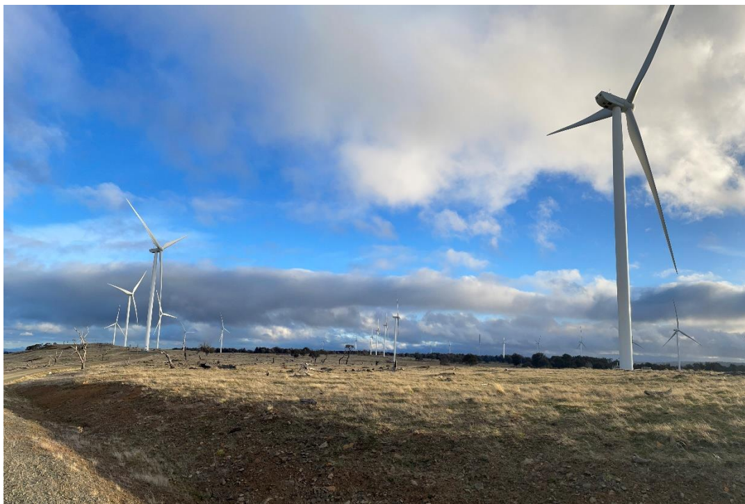
Figure 1.1: Cattle Hill Wind Farm
