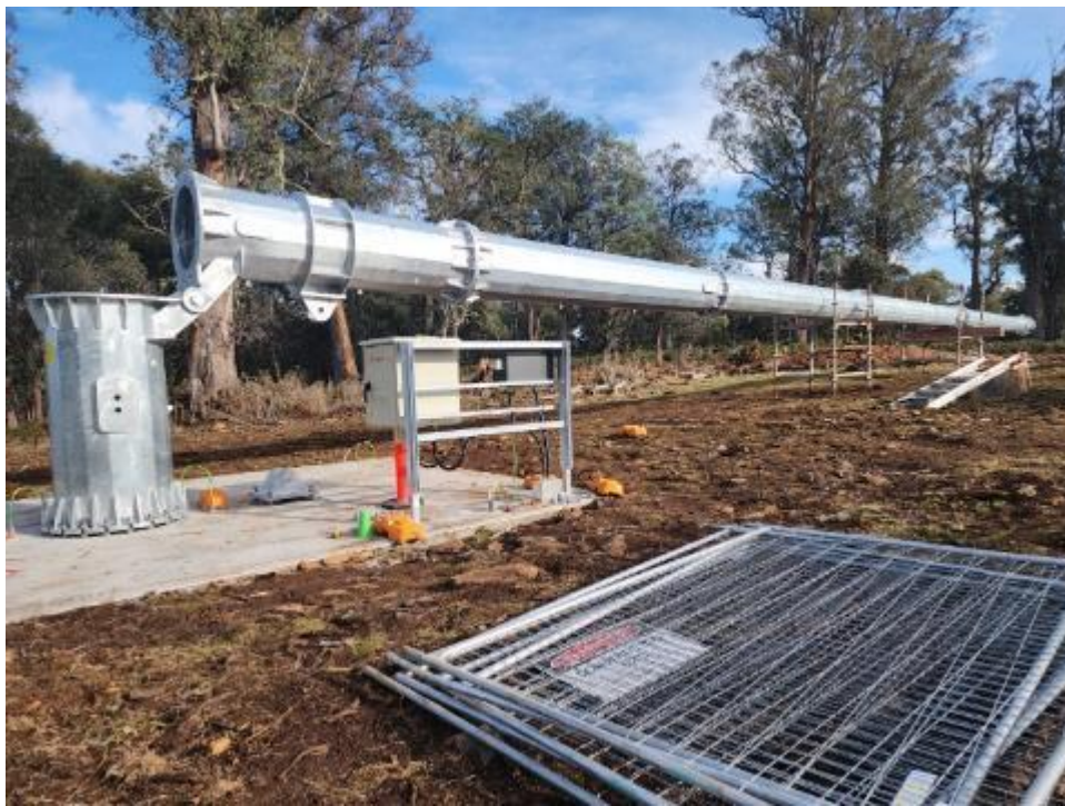
Photograph B2: Foundation and tower pre-lift
