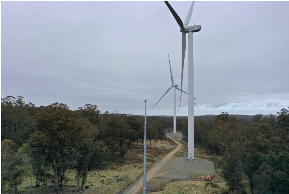
Photograph B1: 30m additional IDF station completes commissioning and commences curtailing turbines (October 2023)
