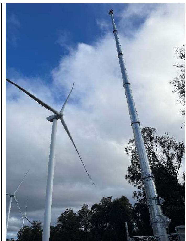
Plate 4.1 – View of IDF 17 30 m tower
